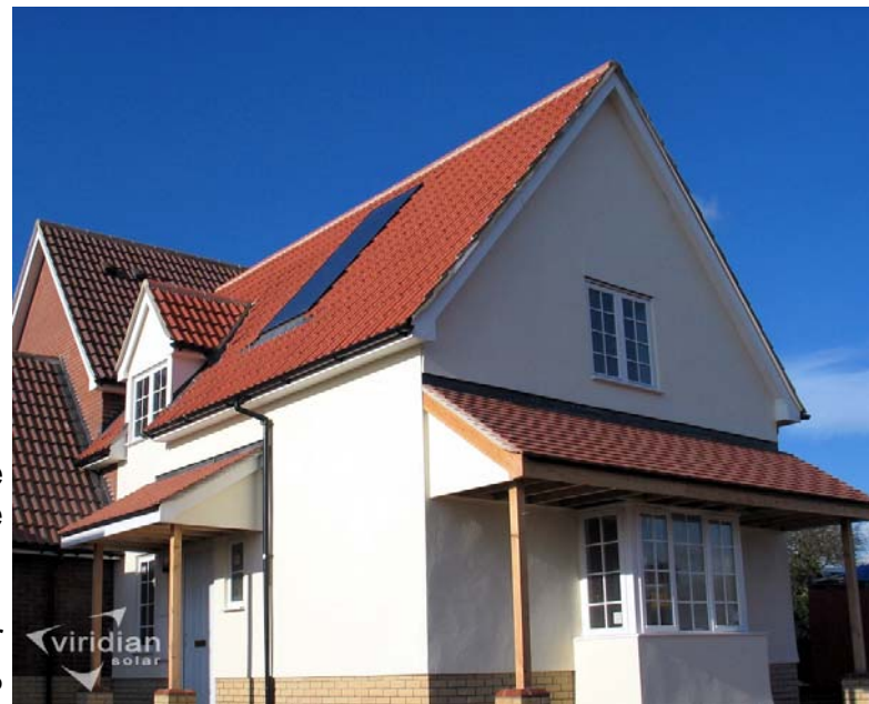
Hastoe Housing Association, Steeple Bumpstead, Haverhill
