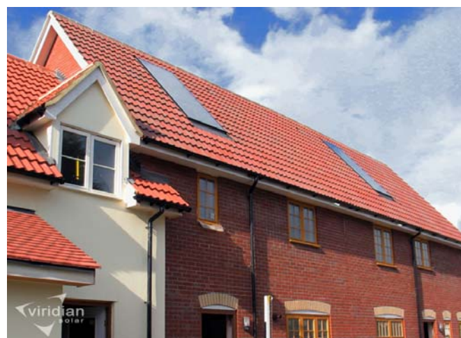
Hastoe Housing Association, Steeple Bumpstead, Haverhill
