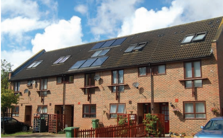
The only outward indication that the middle house in this terrace uses 20% of the energy of its neighbours is the discreet roof-integrated Clearline solar heating panels (lower three) and Clearline PV panels (upper three).
